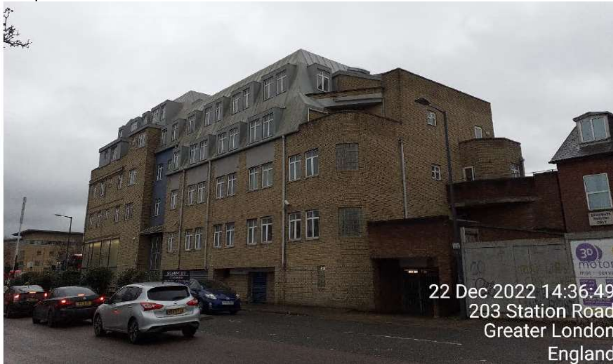
Blue point court to the east:
